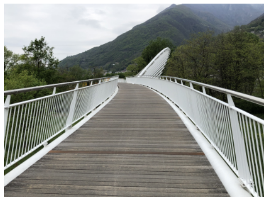
Passerelle in Locarno
